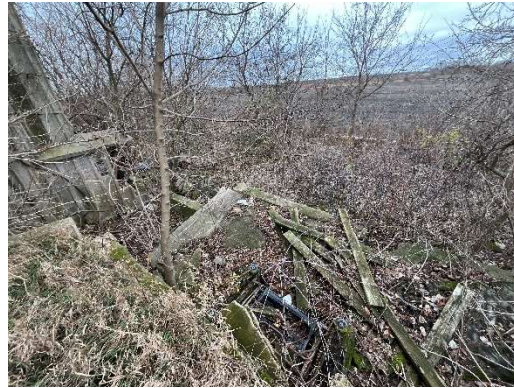
View of Building Remnants Near Dilapidated Silos
