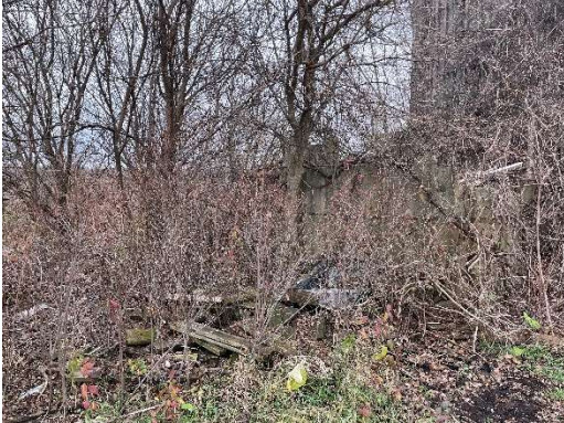
View of Building Remnants Near Dilapidated Silos
