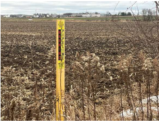
View of Petroleum Pipeline at Northeast Corner of 02-19-200-007
