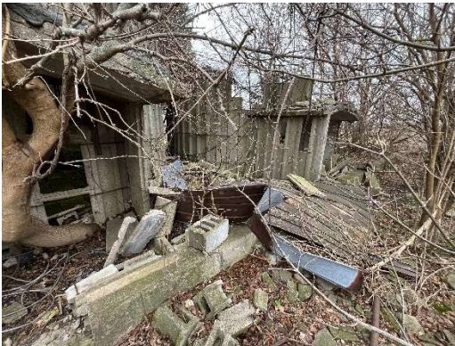
View of Building Remnants Near Dilapidated Silos
