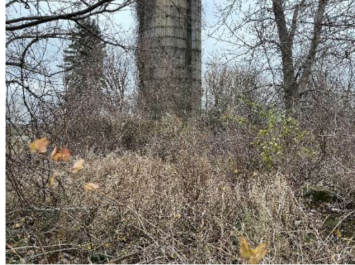
View of Building Foundations Near Dilapidated Silos
