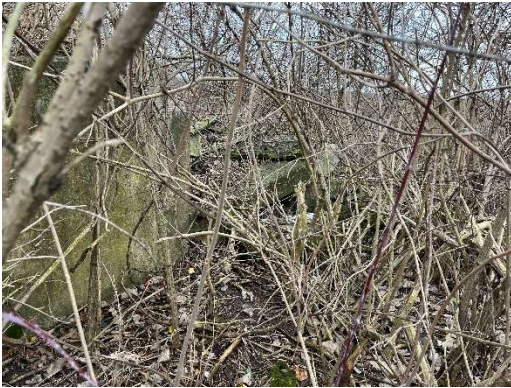
View of Building Foundations Near Dilapidated Silos
