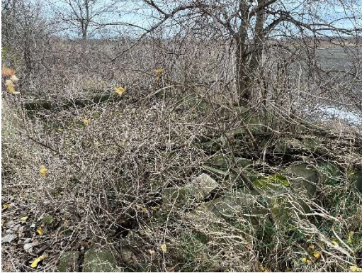
View of Building Foundations Near Dilapidated Silos
